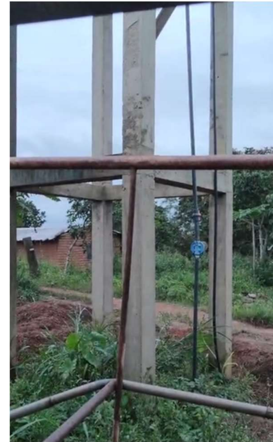
The tank was original supported by a metal structure
